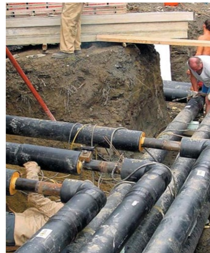
To remove the heat, water flows through the hollow steel rollers, transporting the thermal energy into the pump house via pipelines.
